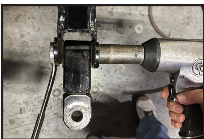
3. Using a 1-1/8" socket and wrench, remove the one (1) bolt attaching the pivot block to the receiver. Remove bolt and washer, set aside to be reinstalled. Discard old pivot block.
