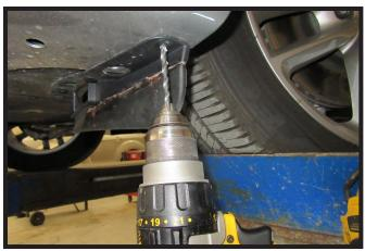
4. Using a 1/4" drill bit, drill out the aluminum pop rivet in front of the tire. Do this on both sides of the vehicle.
