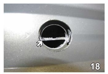
Inside the 1-1/2" drilled hole is a cross piece, which may need to be bent vertically with a pry bar in order to insert 3/8" nut plate. Do this on both sides.
