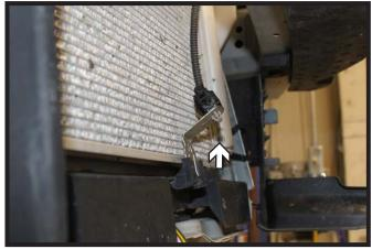
7. If needed bend the temperature sensor up slightly to allow easier baseplate installation.
